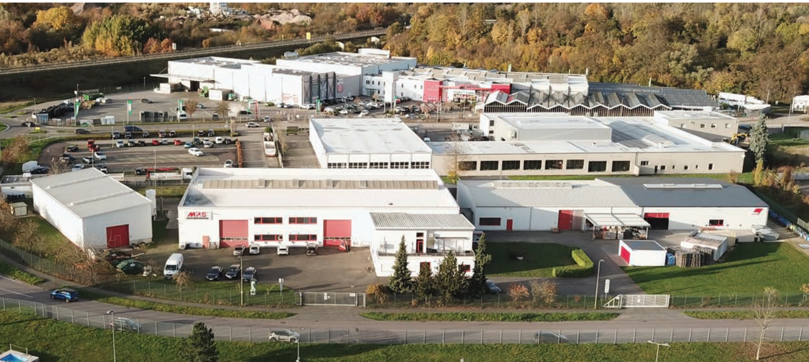
The MPS site in Wasserliesch, Germany
